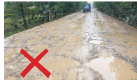
Potholed & Rough Roads
